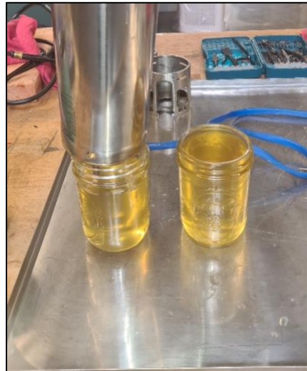
Figure 8: Example of submersible pump motor enclosure being drained into a container for observation.
