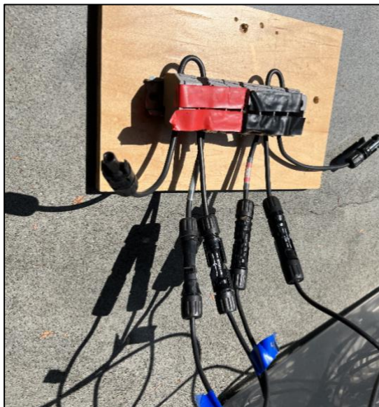
Figure 7. Parallel adapter for PV array circuits that have two parallel strands.
